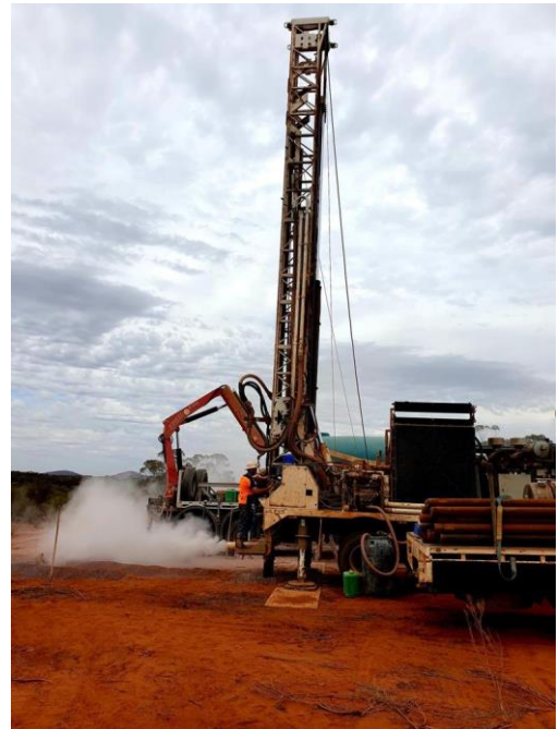
Figure 4. Drilling at Site 3, January 2020.
