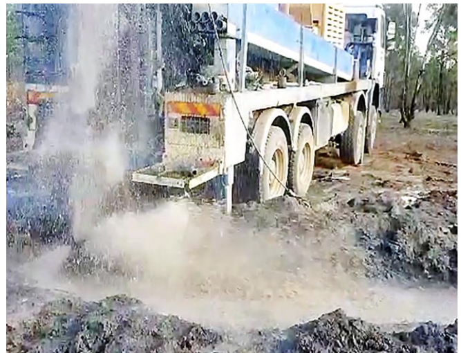
Figure 5. Water flowing from bore during drilling
