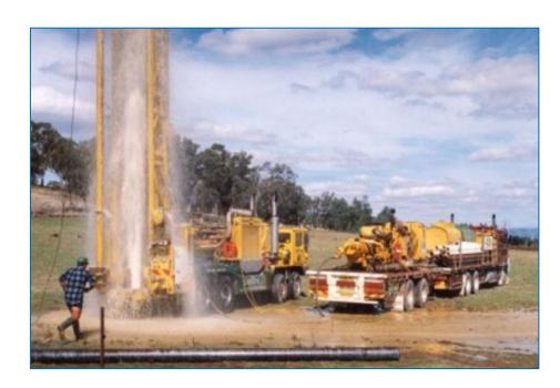
Well drilling costs and effort will vary greatly depending on the location, geology, size, and depth of the well. In some cases, for example, it will require drilling rigs with a capacity to drill through hard rock. Although many bore holes are shallower, the typical depth for a DSW well is 100-200 meters (328-656 feet). AquaterreX can provide and manage the drilling process or work with your preferred drilling contractor.
